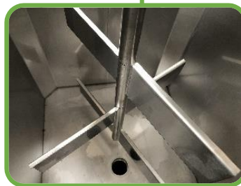
Stainless steel SUS304 Mixing agitator for polymer mixing and prevent coagulation of sludge.
