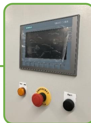
Touch screen control panel with user friendly interface for convenient operation in both automatic and manual function.
