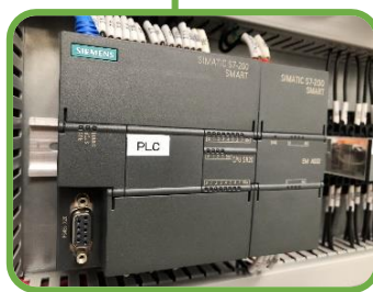
Programmable Logic Controller (PLC) provides flexible operation and overall controlling of machine according to the user needs.
