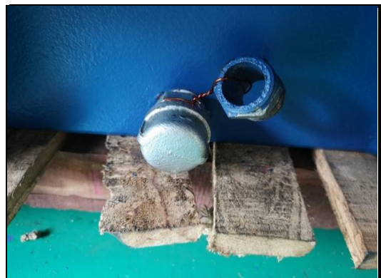
Replace New Nipple Plug
